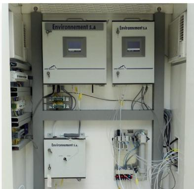
MIR 9000 CLD with the multiplexing system MVS
