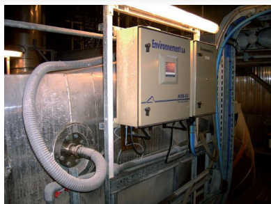
On-stack or close-coupled installation
